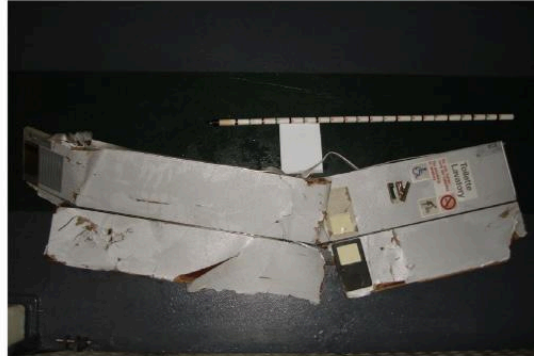
Figure 37: Metallic stiffeners deformed by buckling
