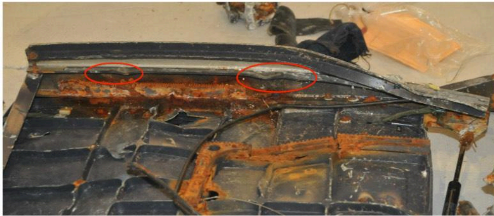
Figure 80: Roller marks on the guidance rail
