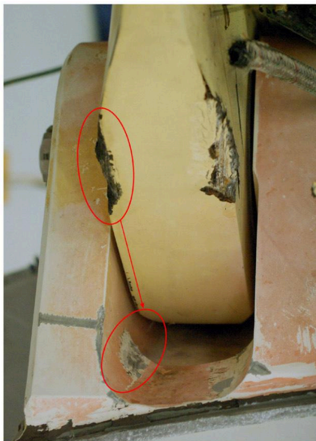
Figure 52: Rear view of the left-hand aft lug: there were marks showing a backwards pivoting of frames 86 and 87
