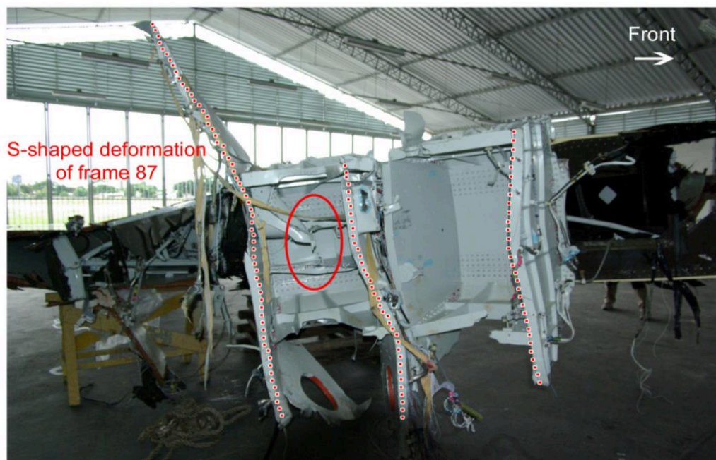
Figure 50: Frames 84 to 87: S-shaped deformation of frame 87, with frames 84 and 85 pushed in backwards; failure of the horizontal stabiliser actuator supports between frames 86 and 87 (red circle)
